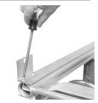
Install screws through both brackets and into each corresponding base rail using a Phillips type screwdriver.
