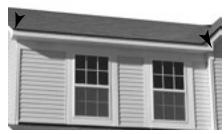
Measure the length of the trim piece. Be sure to add for corner or end laps. If trim piece length exceeds the length of the brake, measure for two pieces and determine best point for overlap.
